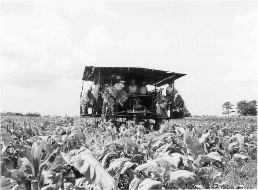
**Figure 15.** A harvesting aid typically used in the 1950s and 1960s that reduced drudgery in harvesting.
