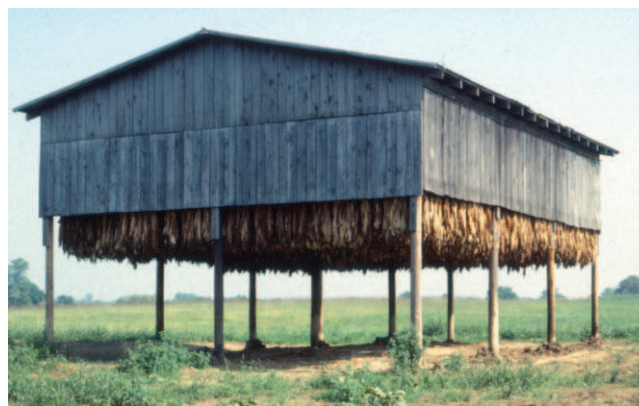
Figure 2. Economy barn of 2-tier height, 2 driveways with slip rails (not shown), partially enclosed side walls, and no doors.
