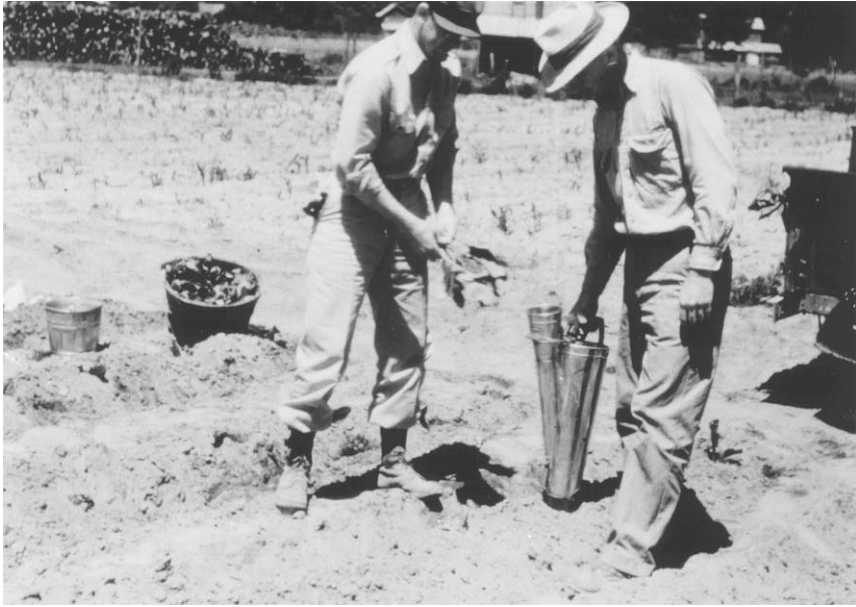
Figure 2. Hand transplanter being used to transplant seedling into a field while adding water to seedling at the same time. Notice that one person operates the transplanter while the other drops the plants.
