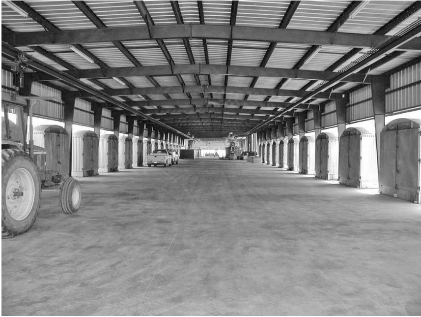
Figure 20. Modern bulk-curing barn complex with large shelter joining units and providing protection from weather for loading and unloading operations.
